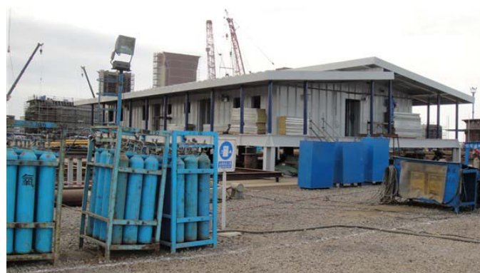
CONTROL BUILDING 外部结构
